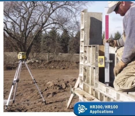
outdoor general construction leveling applications. Combine this versatility with good indoor as well as outdoor visibility, and these receivers are ideal for any general-purpose application.
